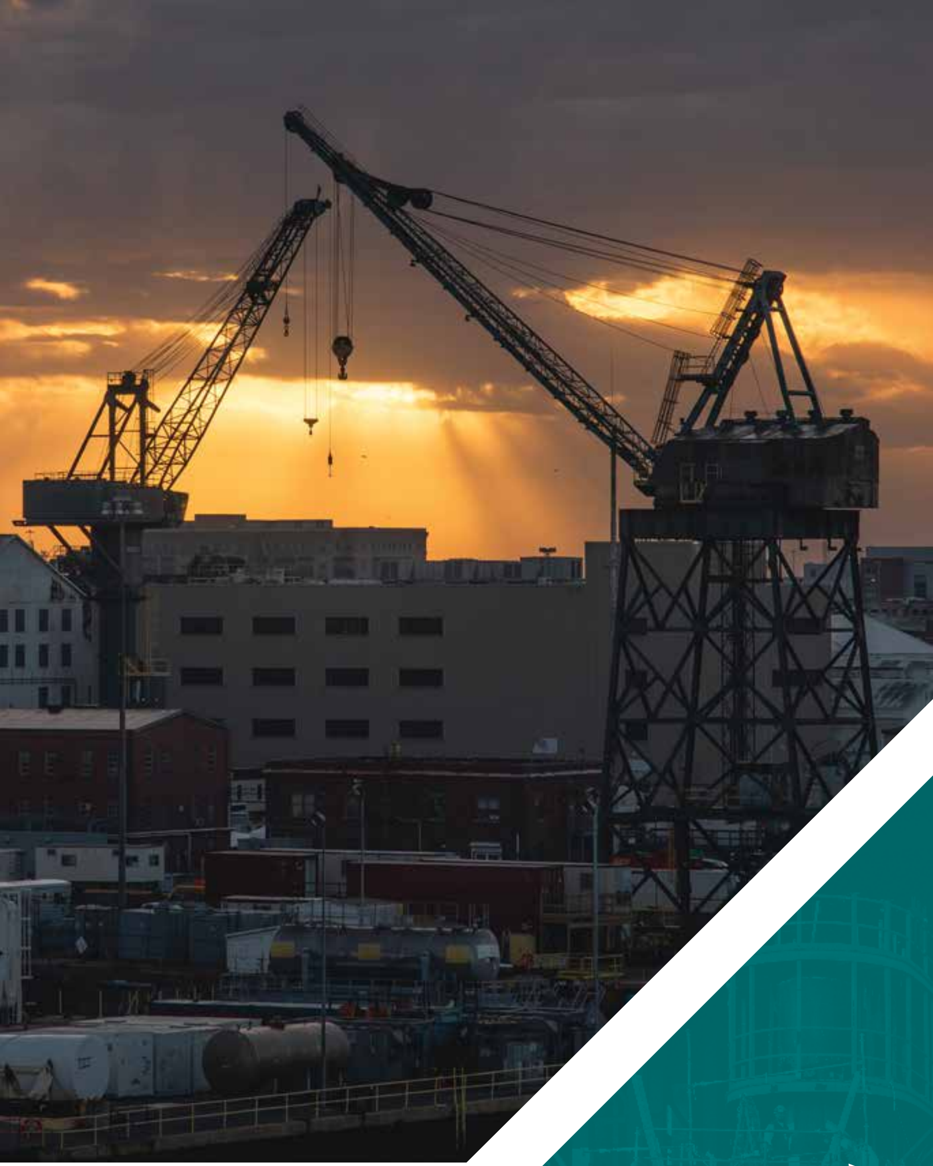
Pictured are two of the more than 500 in-service cranes at Newport News Shipbuilding. These cranes support submarine construction.
