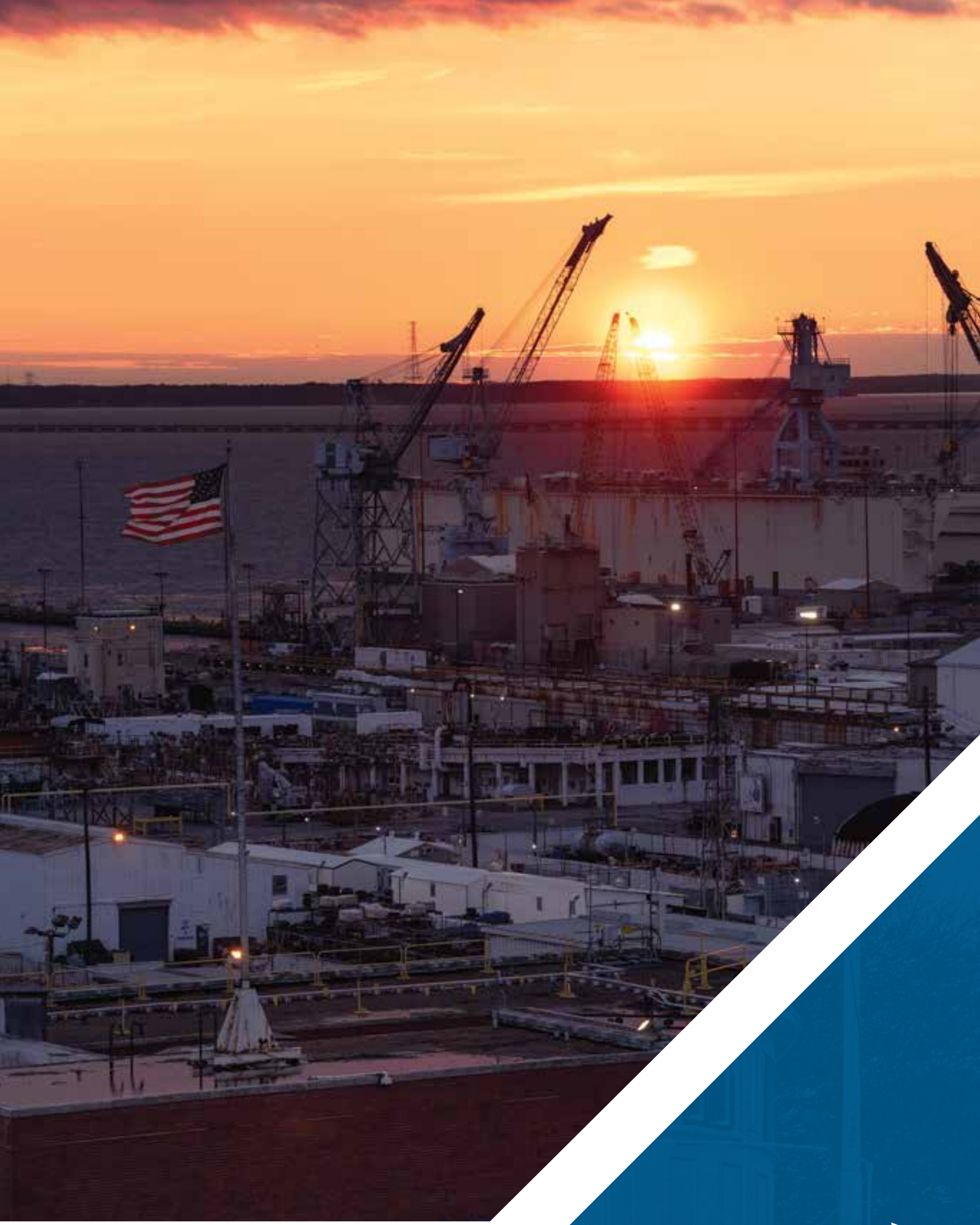
The sun sets over Newport News Shipbuilding's floating dry dock. Built in Japan, the floating dry dock was delivered to the shipyard in 1987 and serves as the launch mechanism for all NNS-built submarines.
